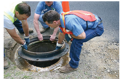
Setting Manhole Frame on Ring
