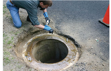
Applying XSEAL to Manhole Ring
