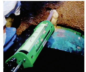
Repaired in Minutes!
