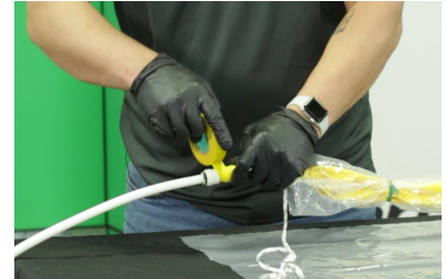
STEP 3 Prepare Packer for Test Install
