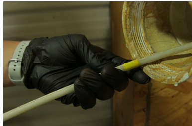
STEP 2 Measure the Repair
