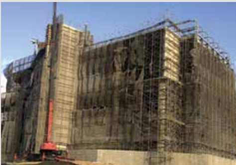
Tung Ho Steel Plant, Taiwan
