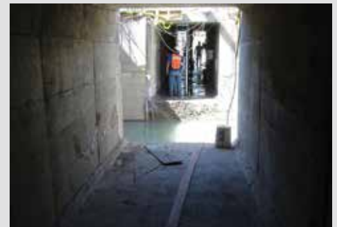
Ensenada International Terminal Tunnel, Mexico
