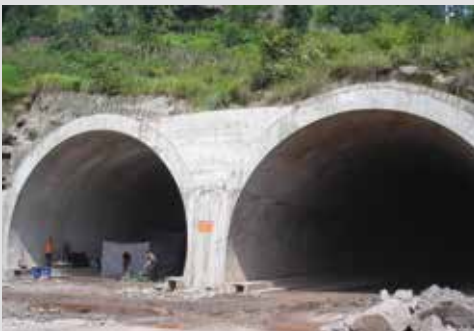
Yunnan Shuima Tunnels, China
