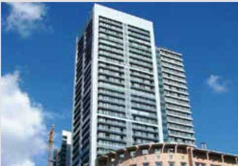
Platinum Tower, Beirut, Lebanon
