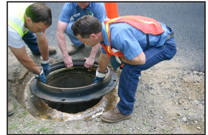
Setting Manhole Frame on Ring
