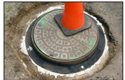
The Job is Finished
