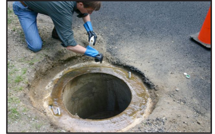
Applying X-Seal to Manhole Ring
